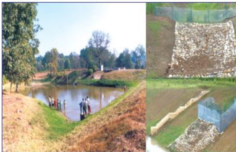
Photo 1: A watershed pond at Selakui research farm showing net lined inlet and outlet at right side
