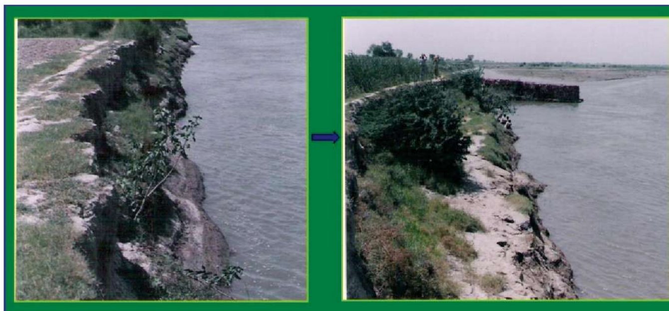
Photo 4.2: Stream bank protection by mechanical measures (Jetties) at Tanaura
