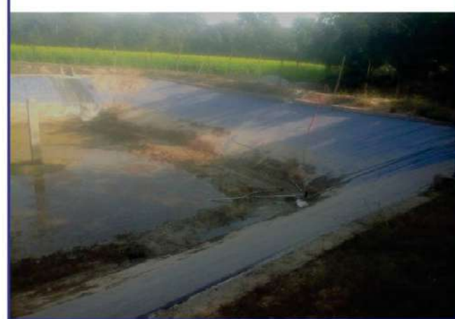
Photo 3.1: Silpaulin lined rain water harvesting pond in reclaimed Yamuna ravines
