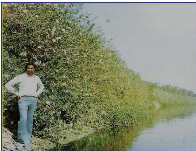
Photo 4.1: Vegetative barrier of Ipomoea carnea to stabilize stream bank
