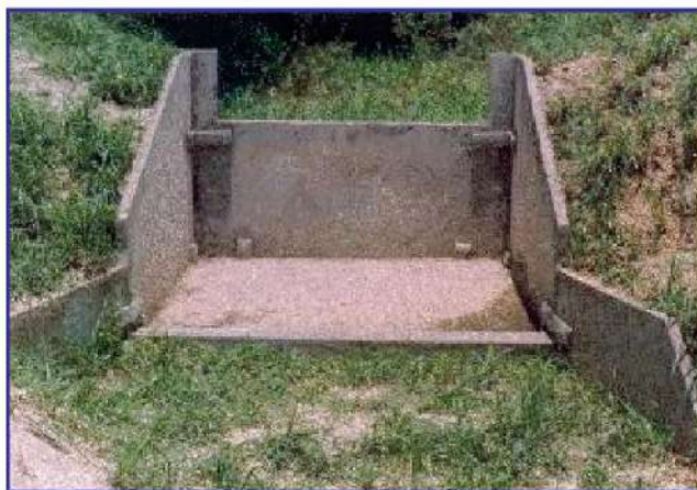
Photo 3.2: Prefabricated drop spillway at site after 13 yrs of installation
