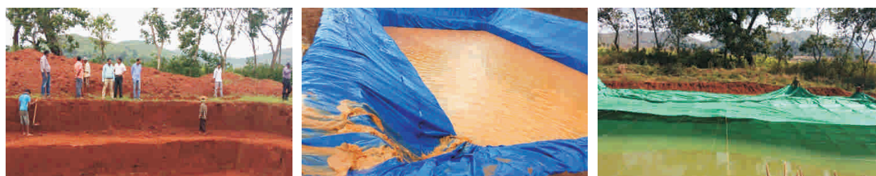
Fig. 21 : Farm pond digging, rainwater harvesting and avoidance of evaporation losses using 25% shade net
