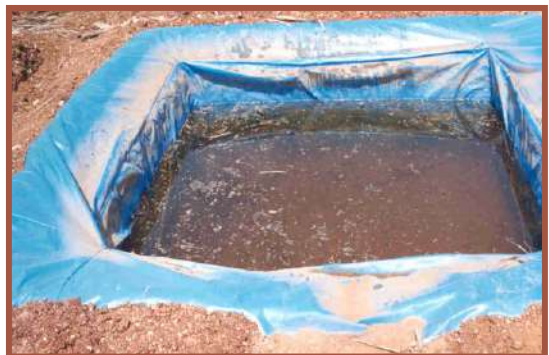
Lined runoff collection pit
