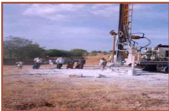
Boring for installing hand pump
