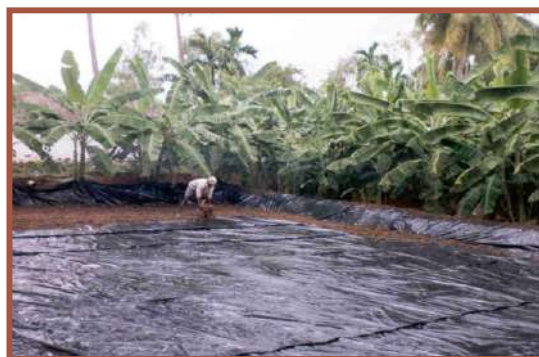
Lining of shallow water storage pond with HDPE sheet
