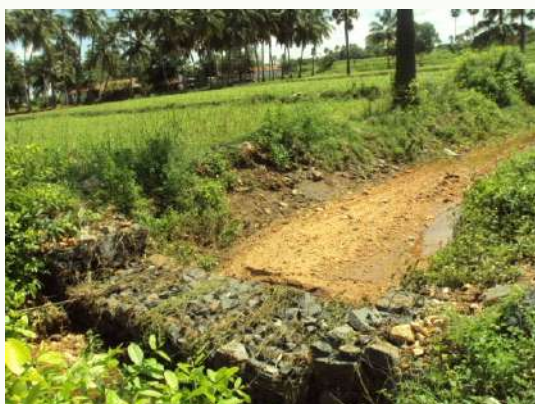
Photo 6: Gabion check dam and RR masonry check dam
