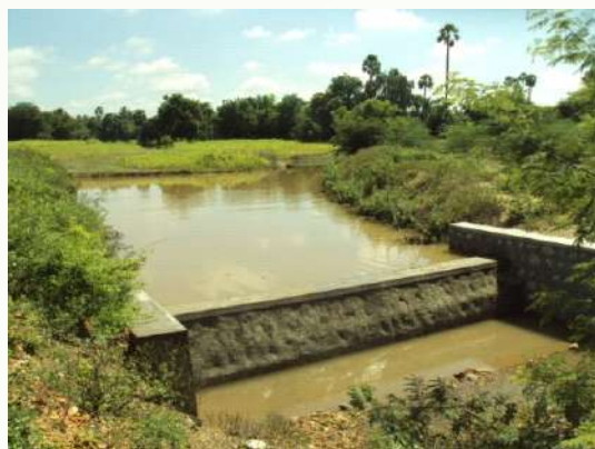
Photo 6: Gabion check dam and RR masonry check dam
