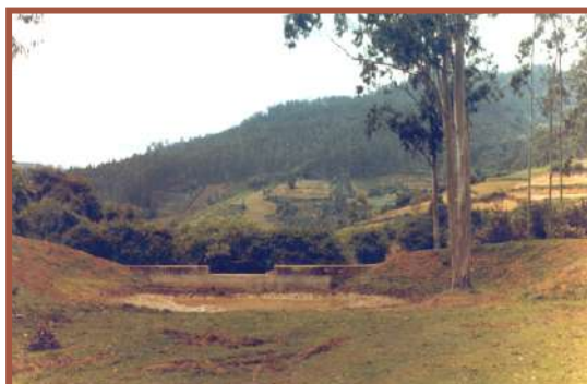
Desilted check dam with side earthen bunds at Kavakadu
