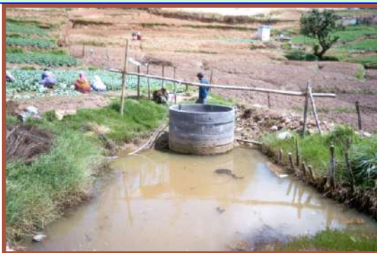
Collection well installed at Kavakadu
