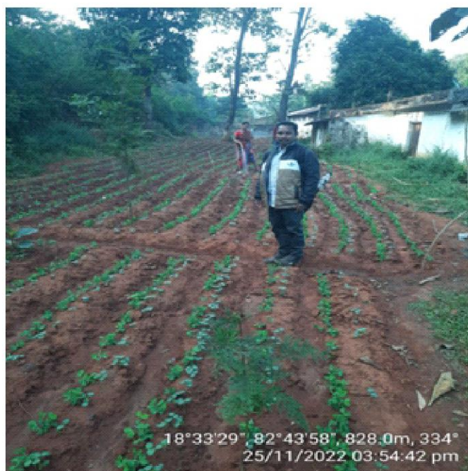
Jhola kundi: A water harvesting technology with solar operated 1 HP pumps along with water distribution system installed/constructed at farmer's field
