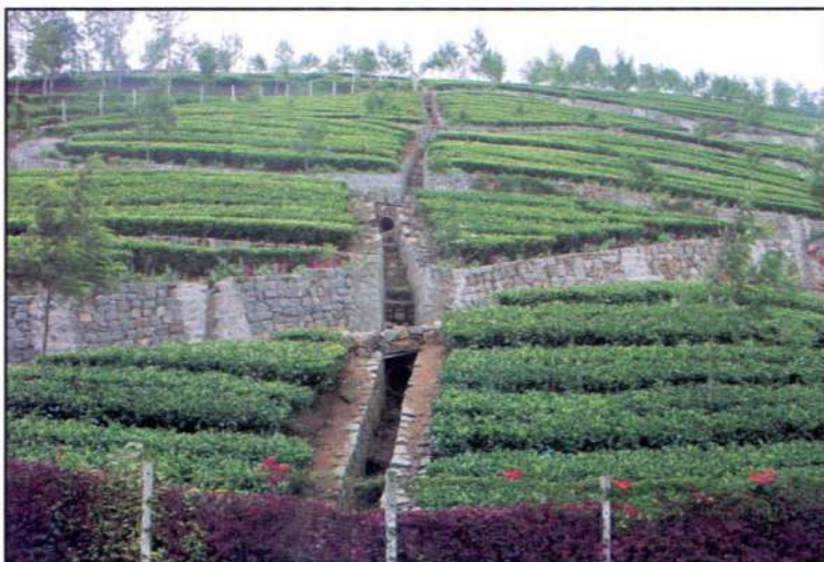
Photo 14 : Vertical drain in tea plantation
