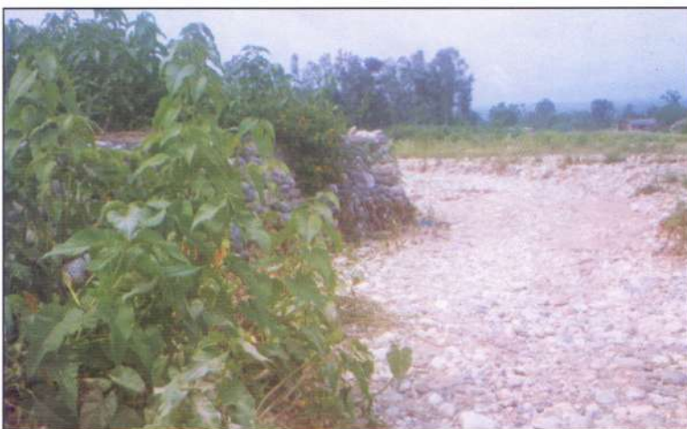
Photo 34 : Vegetative reinforcement of spurs
