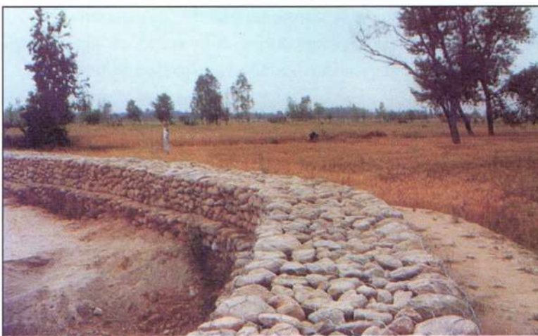
Photo 33 : Agabion protection wall (with steps)
