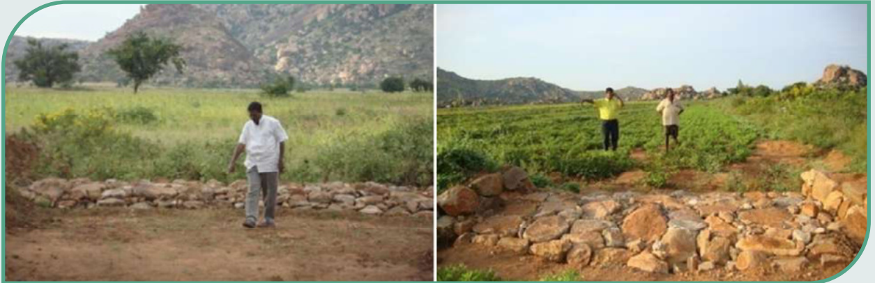
Fig. 5.3. Waste weirs constructed at specified points for safe passage of runoff from fields
