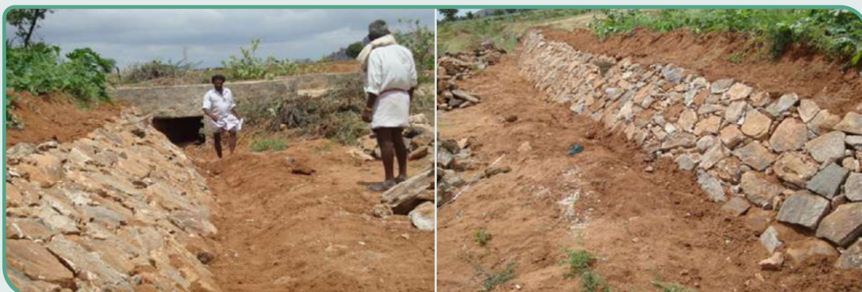
Fig. 5.10. Revetments of cut stones for side walls of water course
