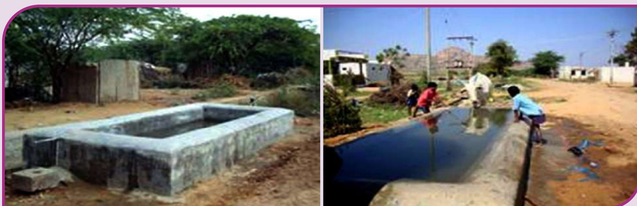
Fig. 3.2. Final view of the Animal water troughs at the Ramasagara watershed
