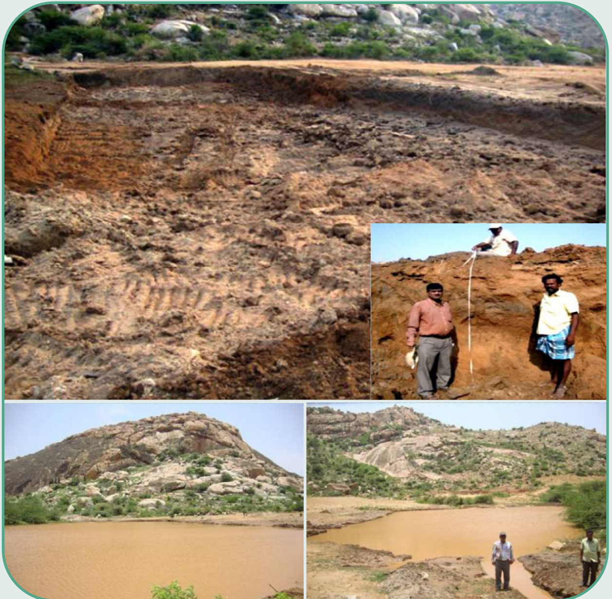
Fig. 5.6. Desilting of percolation tank on the ridge in the upper reach of the watershed
