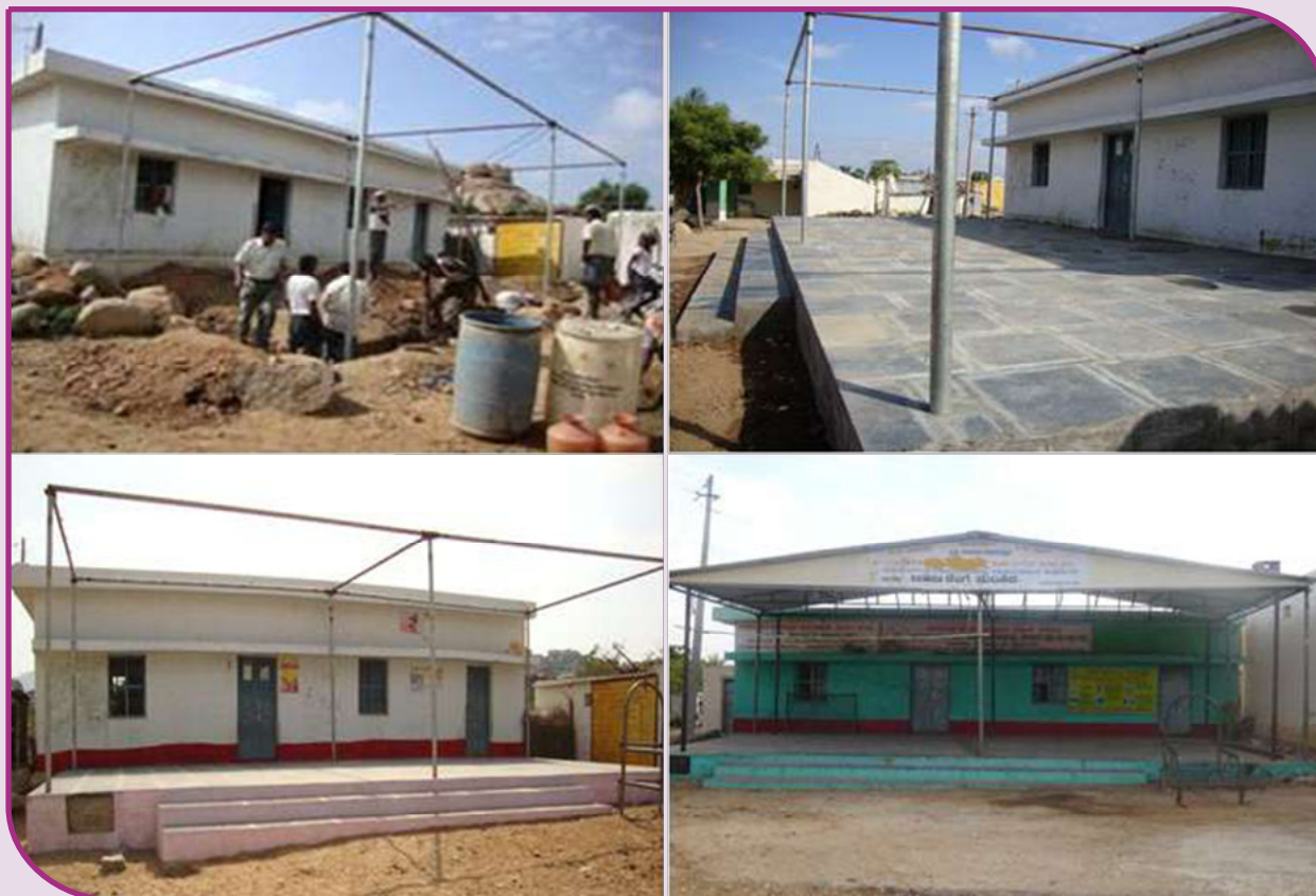
Fig. 3.1. The masonry open-theatre platform
