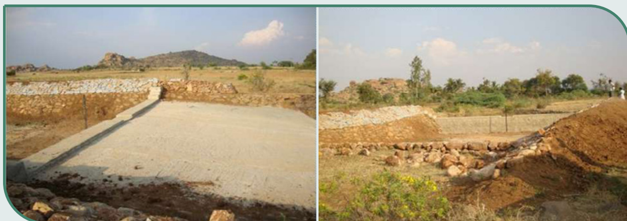
Fig. 5.5. View of the check dam modified as a gauging station
