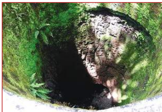
Photo 4.35: Surungam traditional water harvesting system, Kerala
