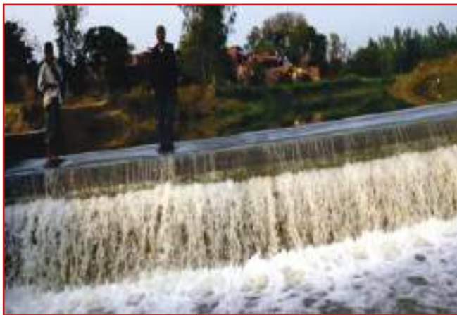
Photo 4.1: Flowing overflow water above weir crest at Sahijana, Lucknow, Uttar Pradesh
