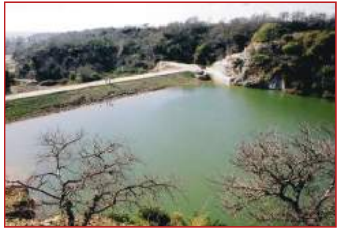
Photo 4.6: Earthen check dam, Sukhomajri, Panchkula, Punjab
