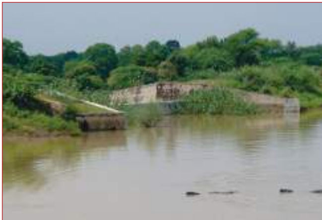
Photo 4.17: Embankment type farm pond with drop structure in Maharashtra
