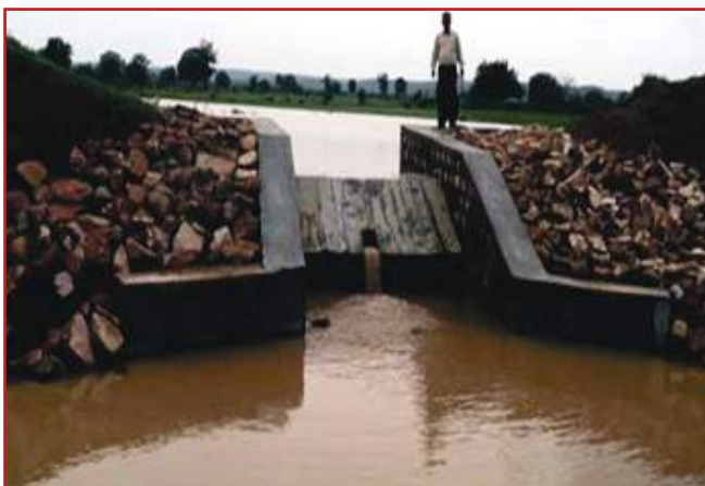
Photo 4.9: Straight drop spillway, Uttar Pradesh
