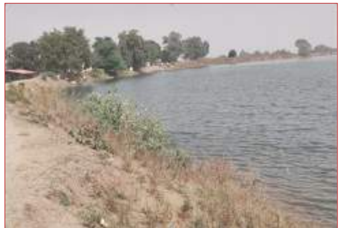
Photo 4.4: A rainwater harvesting tank in district Panna, Madhya Pradesh
