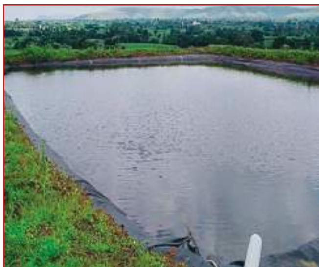
Photo 4.36: Poly lined farm pond, Telengana
