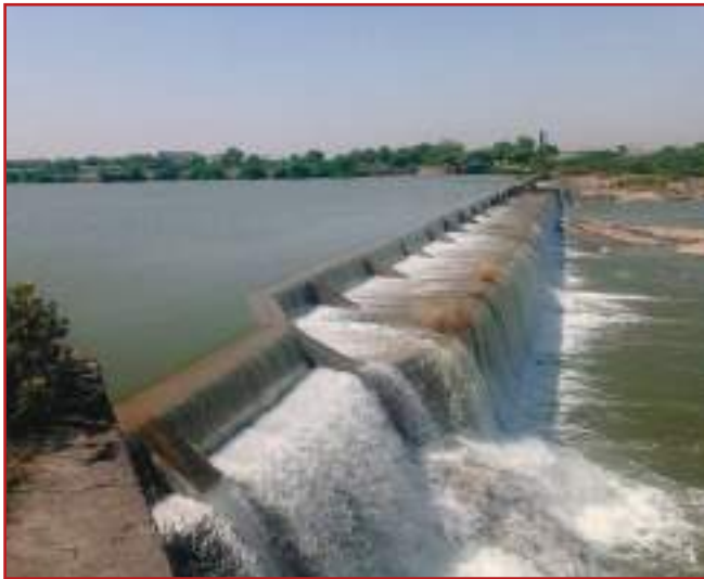
Photo 4.11: Check dam at Panchmahal, Gujarat
