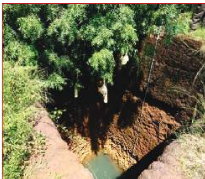
Photo 4.30: Open dug well in Karnataka
