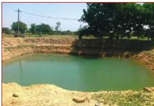
Photo 4.34: Dugout pond - field level water harvesting, Andhra Pradesh
