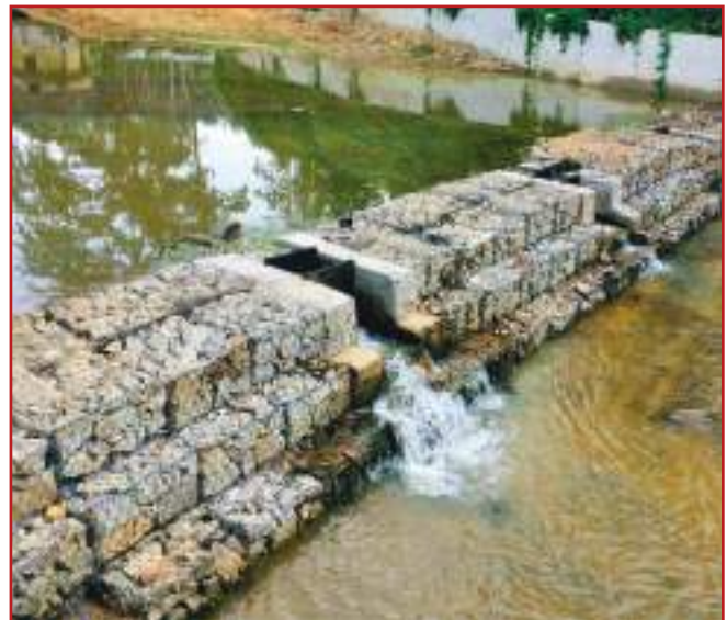
Photo 4.14: Gabion structures for black soil in Maharashtra
