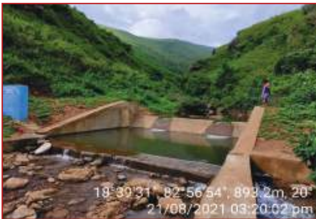
Photo 4.25: Check dam in Southern part of Odisha
