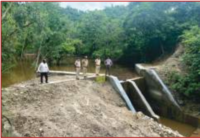
Photo 4.5: Straight drop spillway with Earthen embankment at Ranjeetpur block, Yamuna Nagar, Haryana
