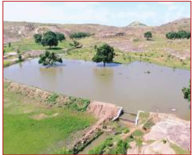
Photo 4.12: Earthen embankment with drop spillway, Gujarat
