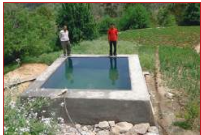
Photo 4.10: Masonry storage tank, Uttar Pradesh
