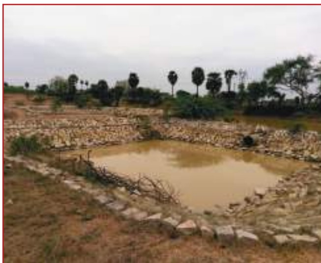
Photo 4.28: Farm pond with dry stone lining in Tamilnadu
