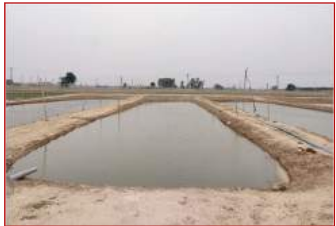
Photo 4.2: A dugout pond for runoff harvesting, Punjab
