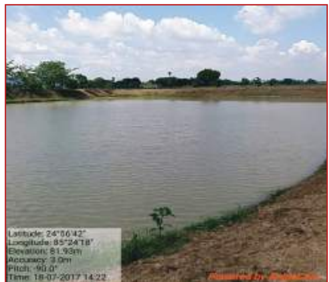
Photo 4.23: Embankment type pond in Bihar
