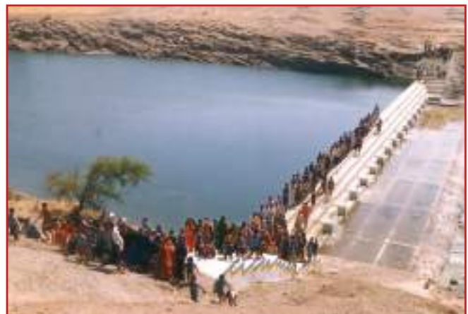
Photo 3.4: Check dam in Maharashtra state
