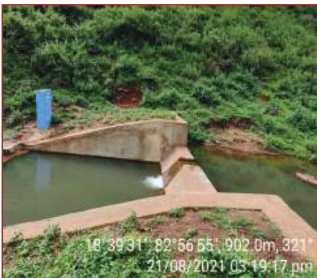
Photo 4.22: Check dam in Southern Odisha
