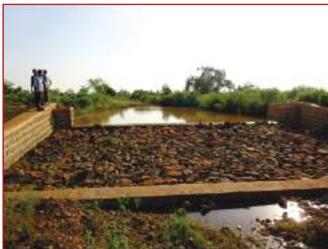
Photo 4.32: Check dam with downstream apron, Raipalli, Bidar Karnataka
