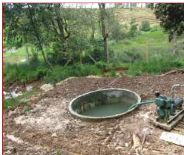
Photo 4.37: Collection well for sub surface water harvesting, Tamil Nadu
