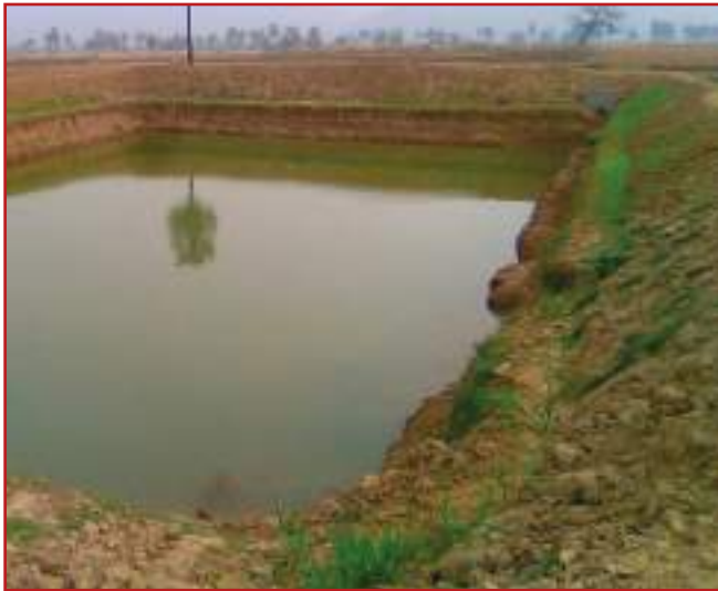
Photo 4.20: Water harvesting pond -dugout in Nawada District of Bihar
