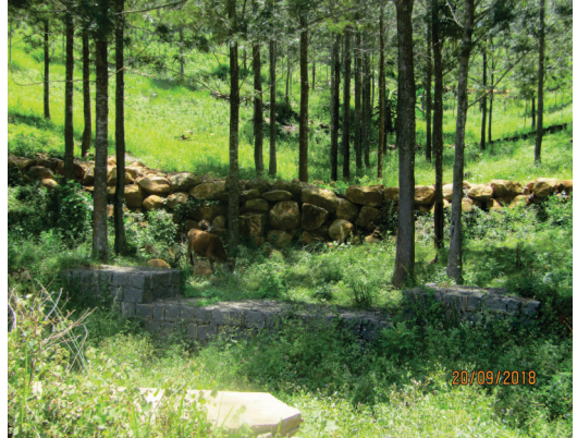
Loose boulder check dam for gully erosion control
