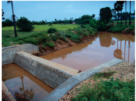
Check dam for water harvesting
