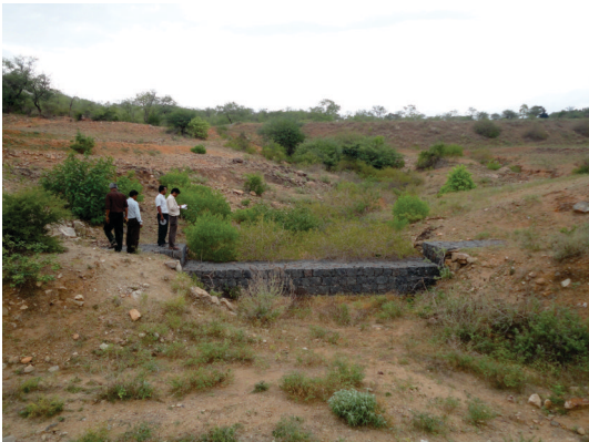
Gabion Check dam for gully erosion control
