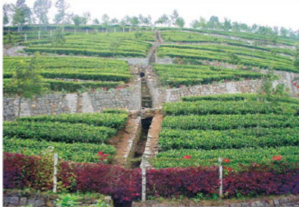
Vertical drain in tea plantation for safe disposal of runoff in the Nilgiri hills
