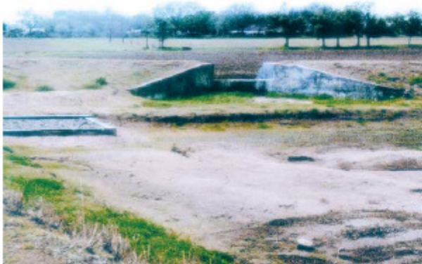
Recharge filter – A cost-effective technology for augmenting groundwater in arable and non-arable lands in the arid and semi-arid regions of Gujarat and Rajasthan
