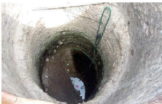
Fig. 5: Status of the water table in the open well before the implementation of runoff filter
