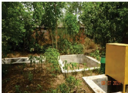
Fig. 3: Downward flow runoff filter in the farmers' field
