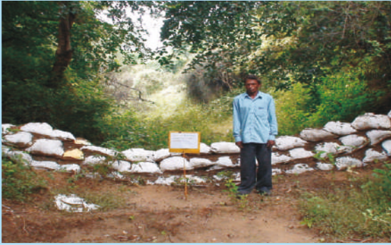
Bori-bund for preventing soil loss from ravine lands and moisture conservation
