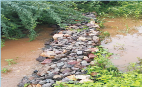
Plastic sheet embedded loose boulder gully plugs for water harvesting and controlling gully erosion in ravine
