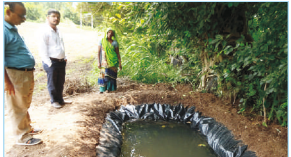
Julkund for rainwater harvesting and supplemental irrigation for plantation establishment in ravines
