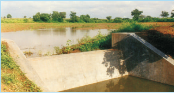
Brick masonry drop cum water harvesting structure
