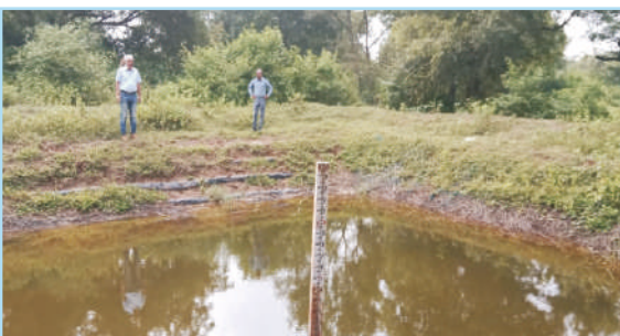
Multi-purpose water harvesting system on the gully head for runoff conservation and recycling of stored water
