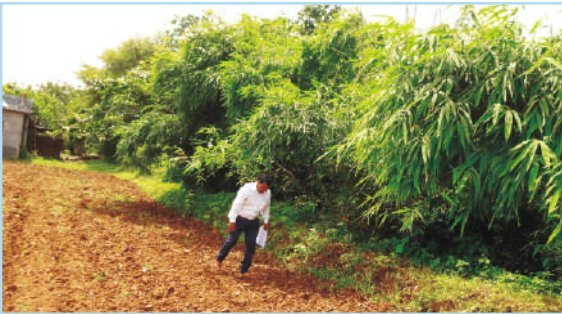
Peripheral bund supported with Bamboo for table land near to gully head in ravines
