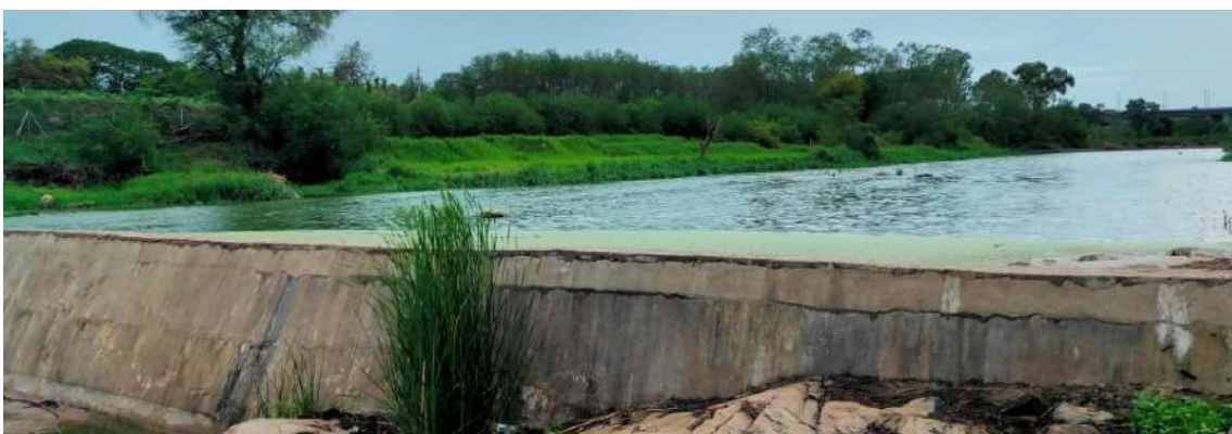
Water harvesting checkdam
