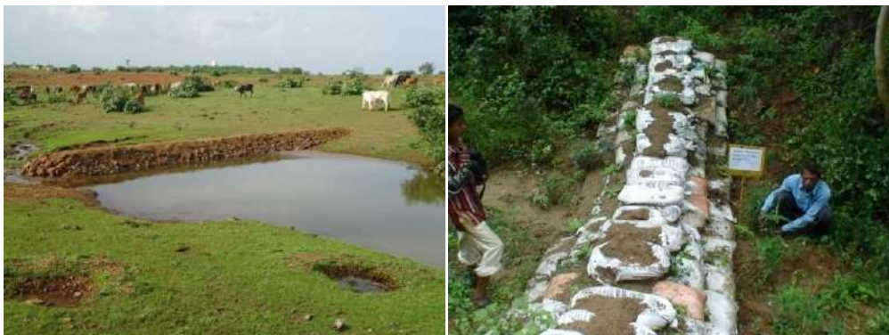
Earthen and bori bunds/sand bag checkdams
