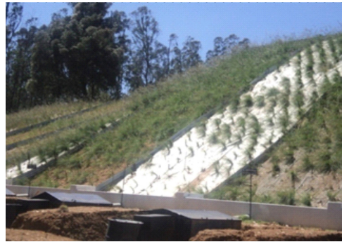
Plate 11. View of the grass establishment during final monitoring period in 60% slope
