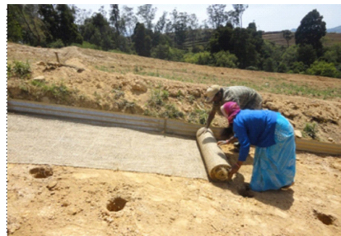
Plate 1. Laying out of three types 500, 600 & 700 GSM of Open Weave Jute Geo-textiles
