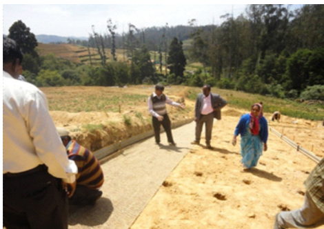
Plate 1. Laying out of three types 500, 600 & 700 GSM of Open Weave Jute Geo-textiles
