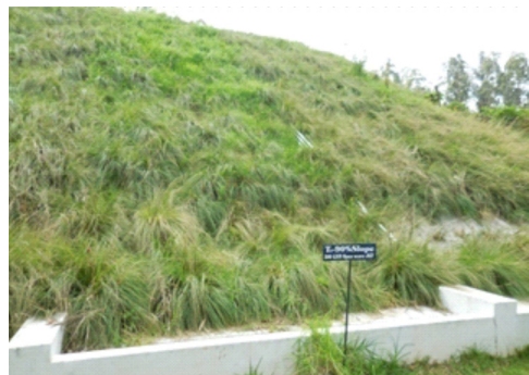
Plate 12. Photographs showing establishment of grass at various stages in 90% slope
