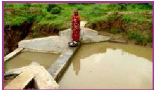
Photo. 9. Check dams constructed for drainage line treatment
