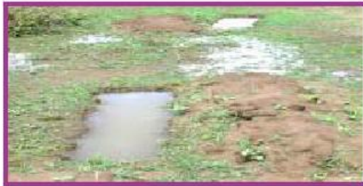
Photo. 6. Staggered contour trenches
