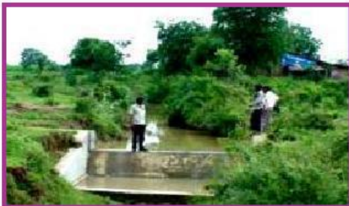
Photo. 9. Check dams constructed for drainage line treatment
