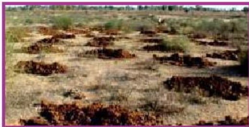
Photo. 6. Staggered contour trenches
