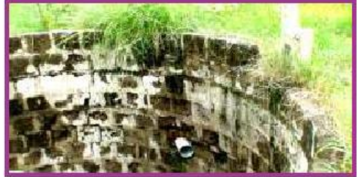
Photo. 12. Recharge filter in arable land
