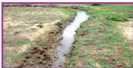
Photo. 7. Continuous contour trenches
