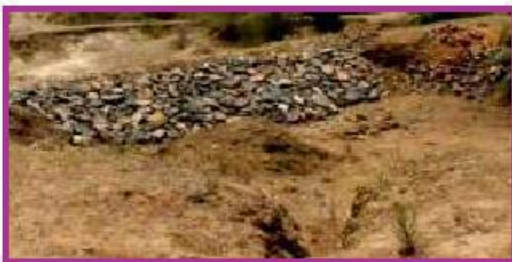
Photo. 8. Gully plug structures in drainage line
