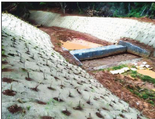
Gully erosion control by geo jute with grass planting
