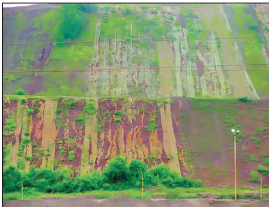
Geo jute cover with grass planting in mine spoiled areas
