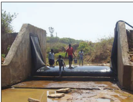
Rubber check dam for seasonal water storage
