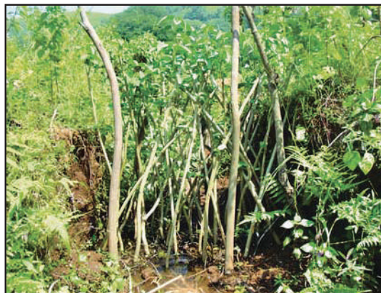
Live check dam for erosion control
