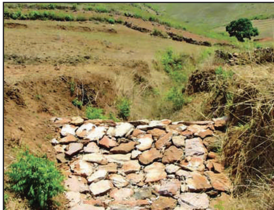
Loose boulder check dam
