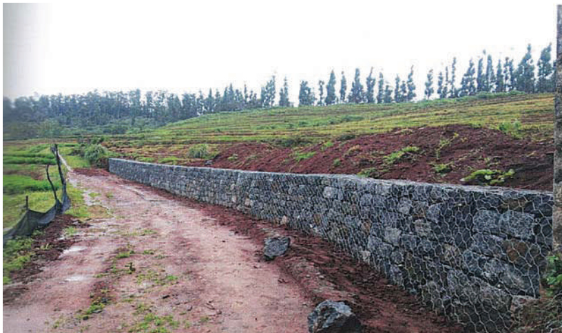
Gabion retaining wall
