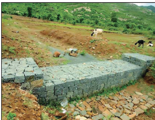
Gabion check dam
