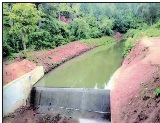
Masonry check dam
