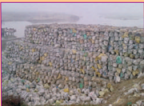
Katta-Crate Technology: A Cost Effective Measure for Rehabilitation of Torrents and Minespoil Areas
