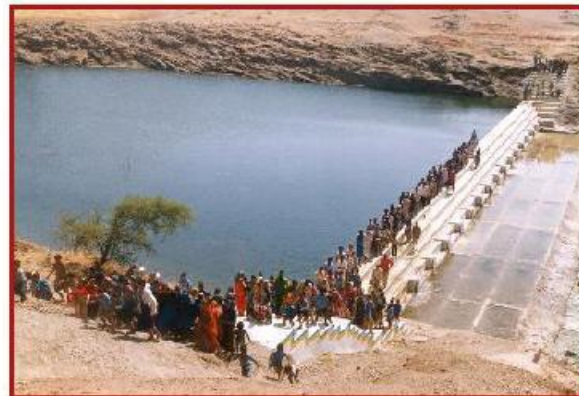
Photo 3.4: Check dam in Maharashtra state
