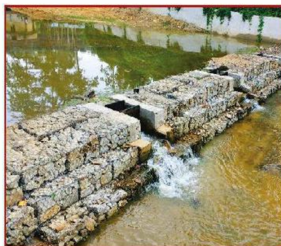
Photo 4.14: Gabion structures for black soil in Maharashtra
