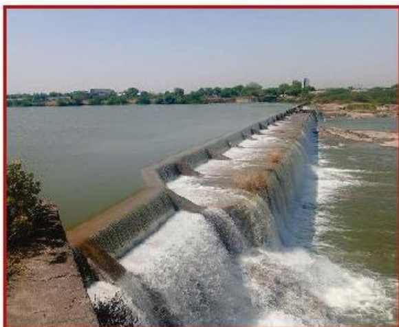
Photo 4.11: Check dam at Panchmahal, Gujarat
