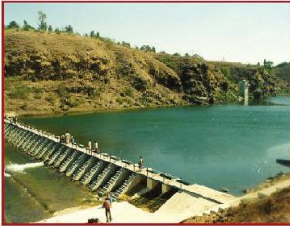
Photo 4.15: Check dam with sluice gate for flow regulation, Dahod, Gujarat
