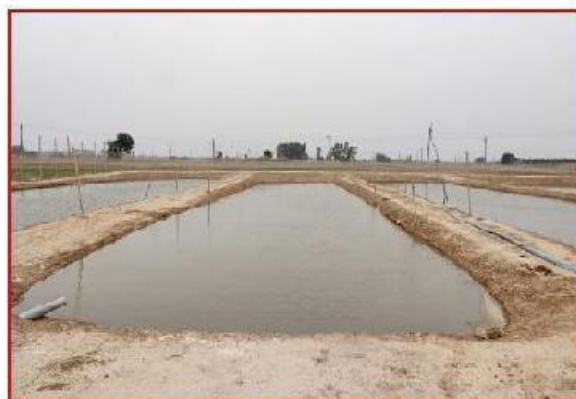
Photo 4.2: A dugout pond for runoff harvesting, Punjab
