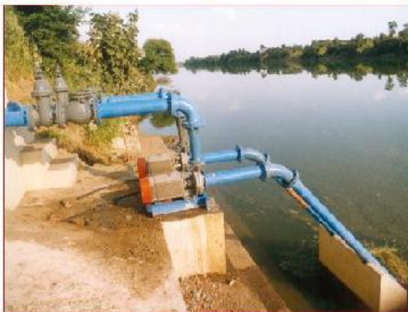
Photo 4.19: Lift irrigation with check dam at Dahod, Gujarat
