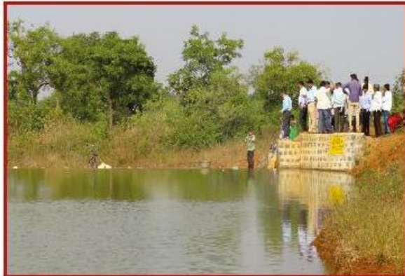
Photo 3.1: Check dam at Raipalli-2 micro watershed in Bidar District of Karnataka
