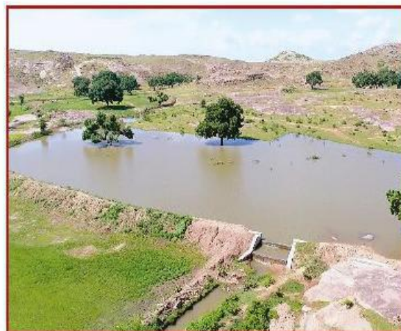
Photo 4.12: Earthen embankment with drop spillway, Gujarat
