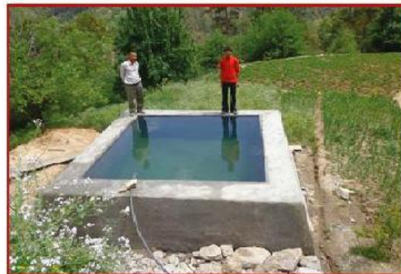
Photo 4.10: Masonry storage tank, Uttar Pradesh
