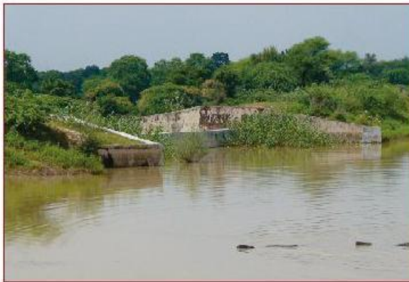
Photo 4.17: Embankment type farm pond with drop structure in Maharashtra
