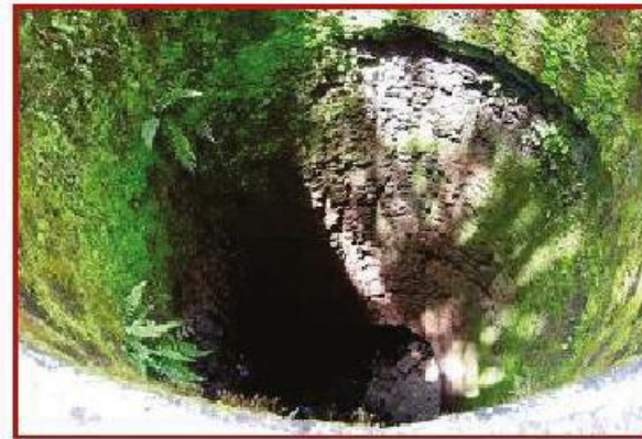
Photo 4.35: Surungam traditional water harvesting system, Kerala
