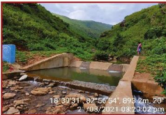
Photo 4.25: Check dam in Southern part of Odisha
