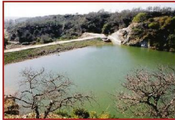
Photo 4.6: Earthen check dam, Sukhomajri, Panchkula, Punjab
