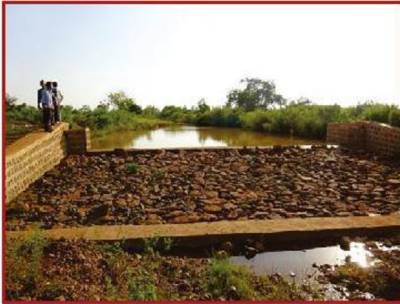
Photo 4.32: Check dam with downstream apron, Raipalli, Bidar Karnataka
