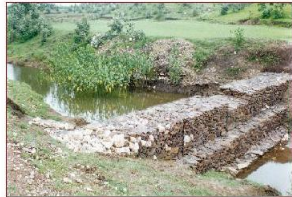
Photo 4.18: Gabion structures for black soil
