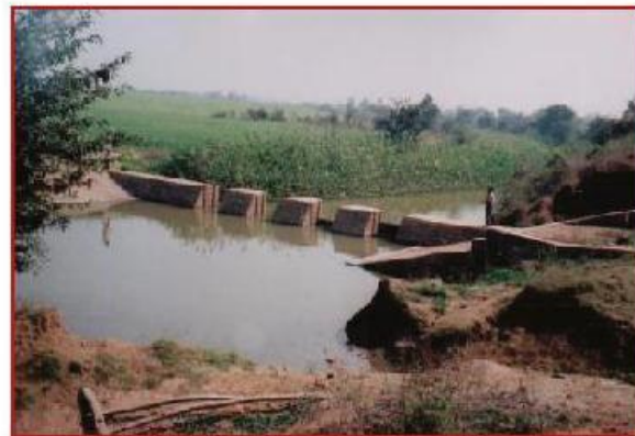
Photo 4.8: A stop dam at Akoda Nadi, Khairoda, district Guna, Madhya Pradesh
