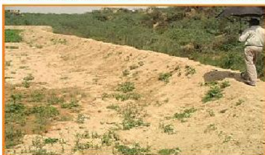
Fig. 3. Peripheral bund for reclamation of shallow ravines
