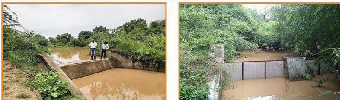
Fig. 7. Composite check dam on gully for reclamation of medium and deep ravine
