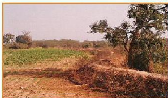
Fig. 3. Peripheral bund for reclamation of shallow ravines
