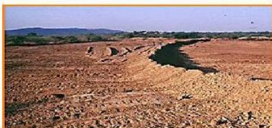
Fig. 4. Contour bund for reclamation of shallow ravine
