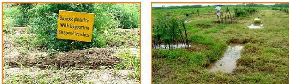
Fig. 10. Trenching for reclamation of medium and deep ravine
