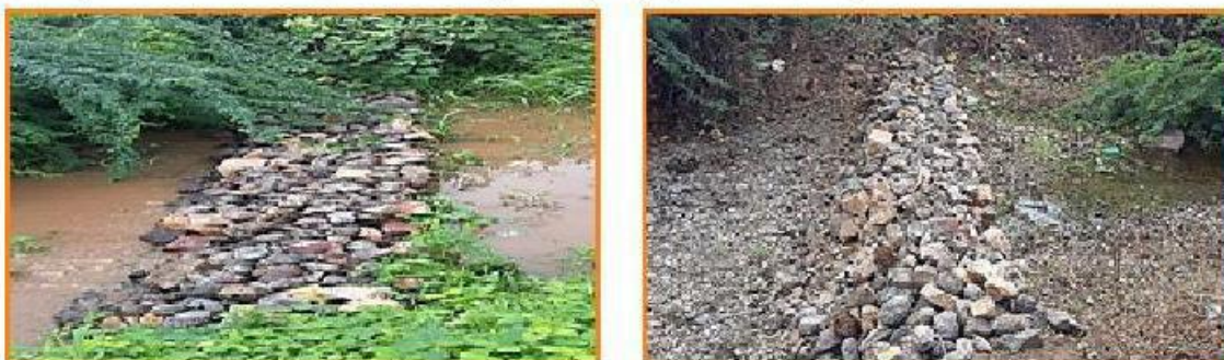
Fig. 8. Gully plugs for reclamation of medium and deep ravine
