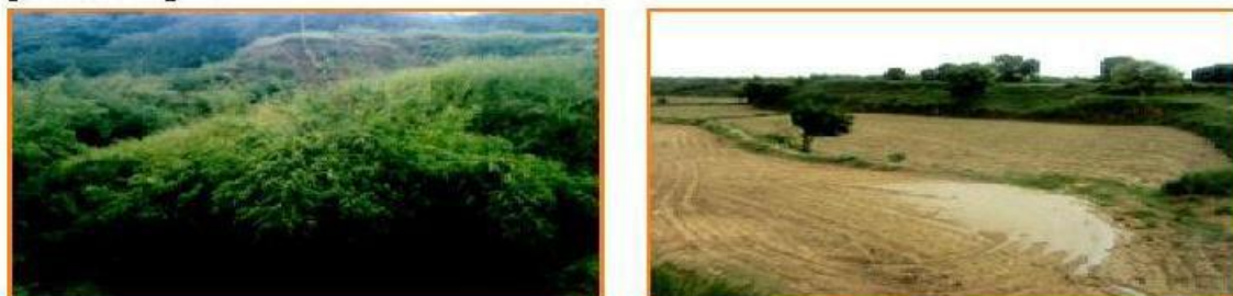
Fig. 15. Conservation measures for development of ravine land
