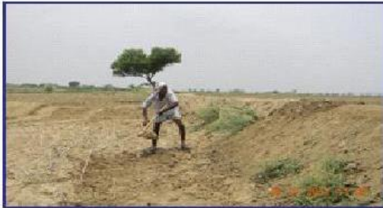
Photo 11: Construction of bund in watershed
