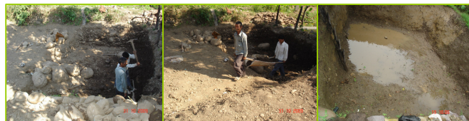
Construction of new ponds for fish farming by motivated farmers continues
