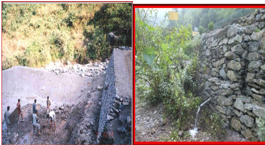
Photo 3. Strategic pond construction and outlet for subsurface flow
