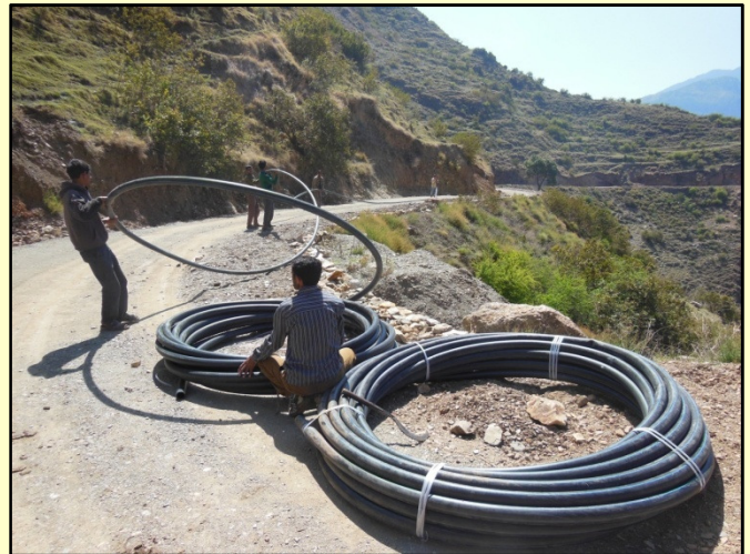
Activity of HDPE pipe laying in Attal Village
